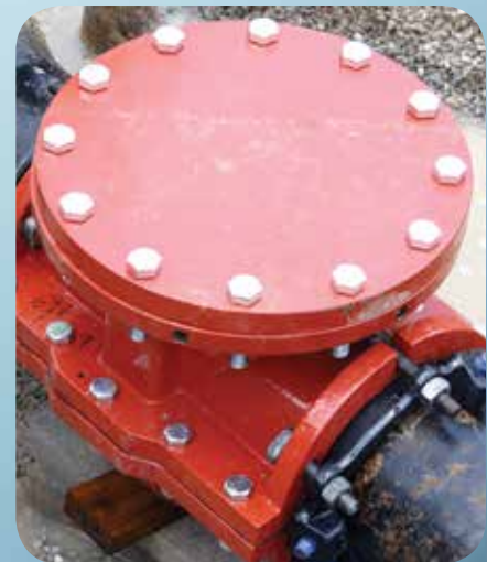
Blind flange installed.
