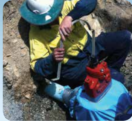
An InsertValve installation under full line pressure.
